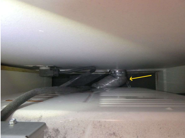
Laundry closet (behind dryer)
