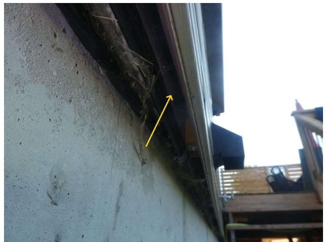
Exterior siding (view from below)
