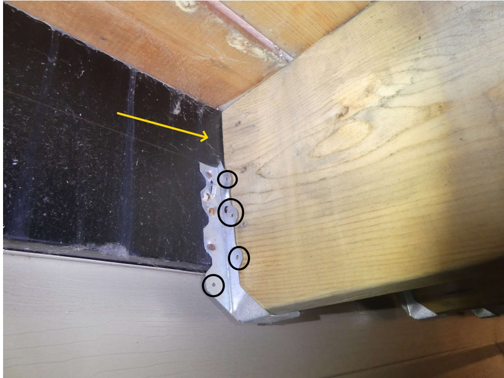
Below rear balcony
