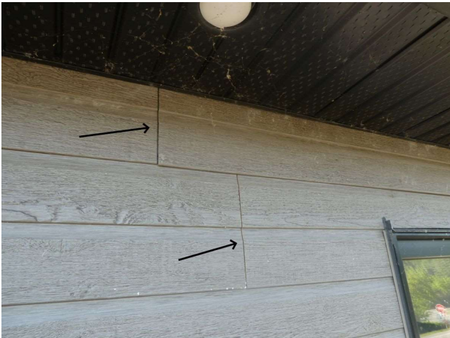
Front facade (above garage)
