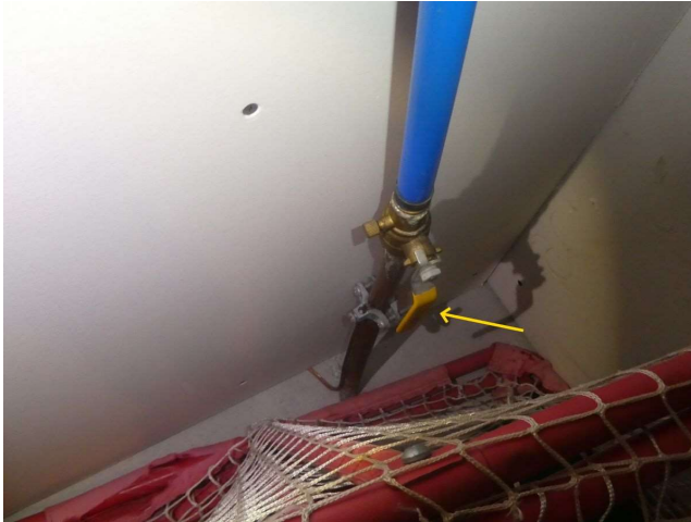
Basement (sump pit room)
