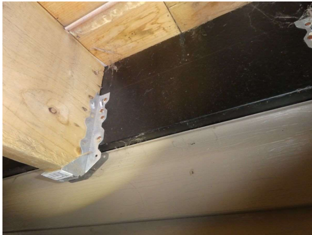
Below rear balcony
