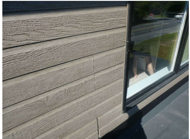
Front facade (above garage)
