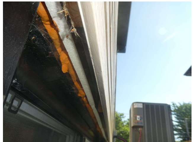
Left facade (view from below)
