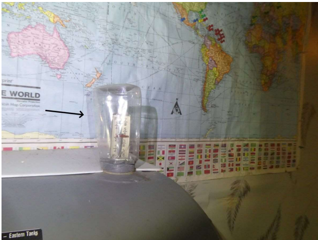
Basement (mechanical room)
