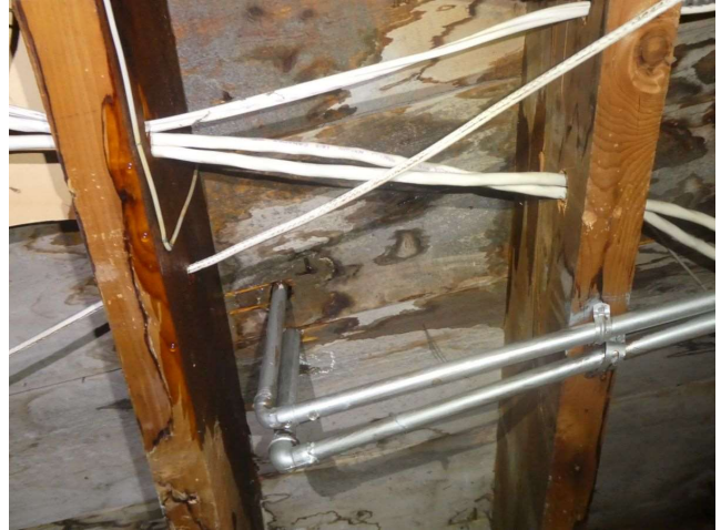
Basement (mechanical room)
