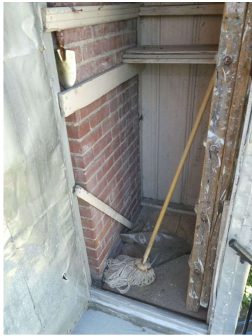
Rear balcony (second floor)
