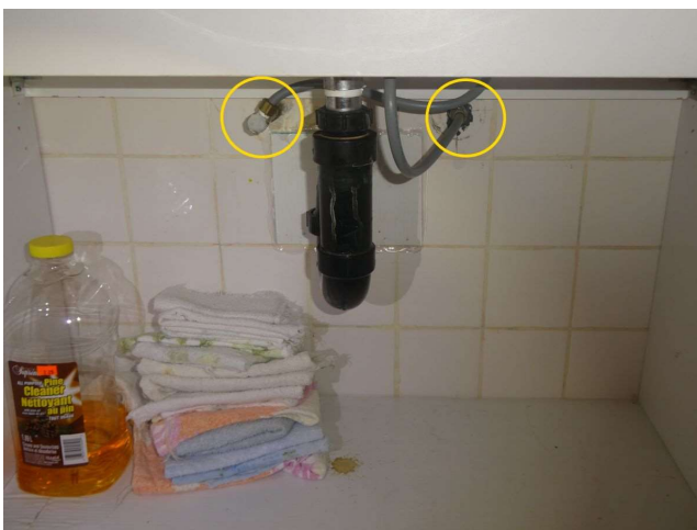
ground floor washroom
