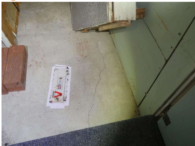
Below basement staircase
