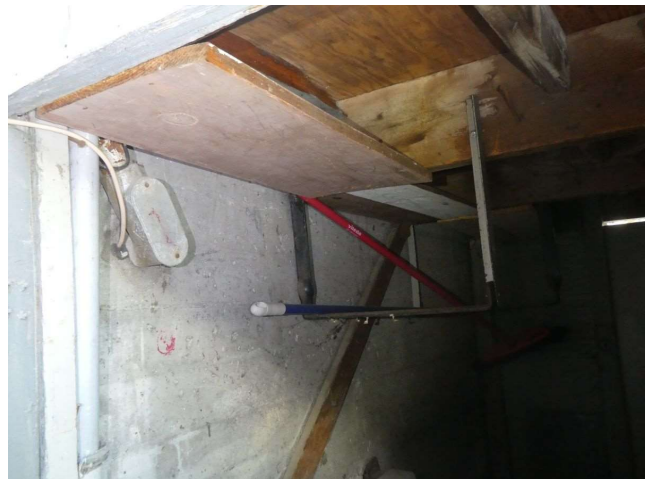
Below rear balcony
