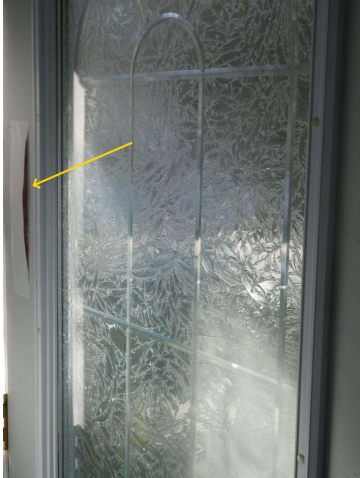
Front door leading to second floor
