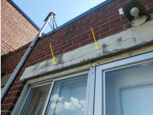
Rear facade (second floor balcony)
