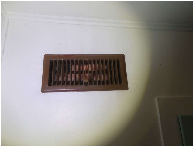
Basement (front room)
