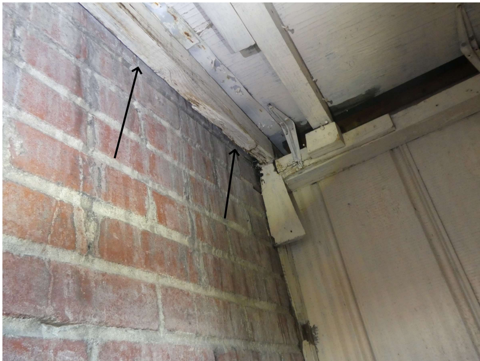
Rear balcony (second floor)
