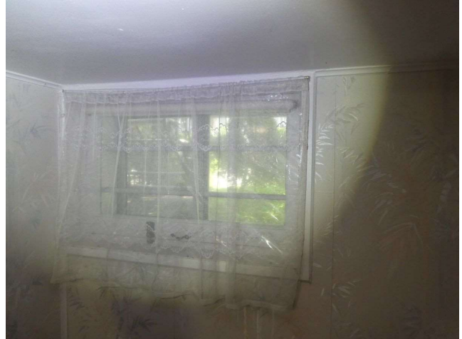
Basement (front room)
