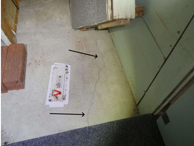
Below basement staircase
