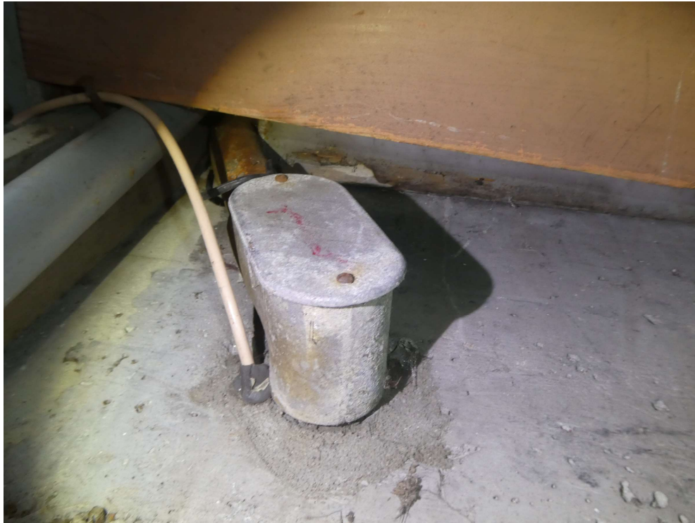
Below rear balcony
