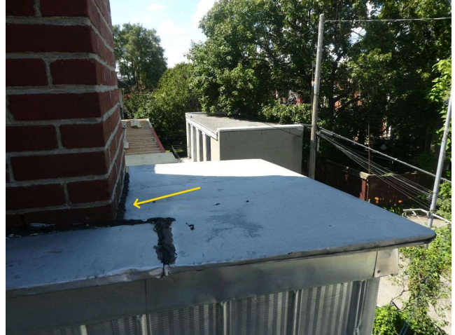
Rear balcony (second floor)
