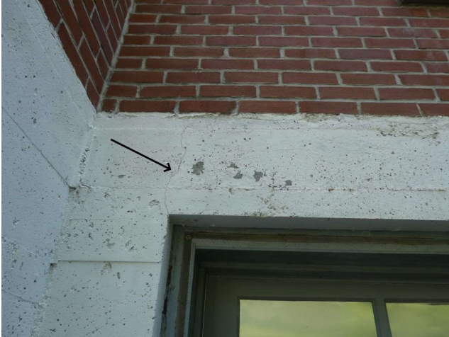
Rear facade (above garage door opening)
