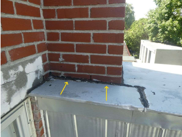
Rear balcony (second floor)
