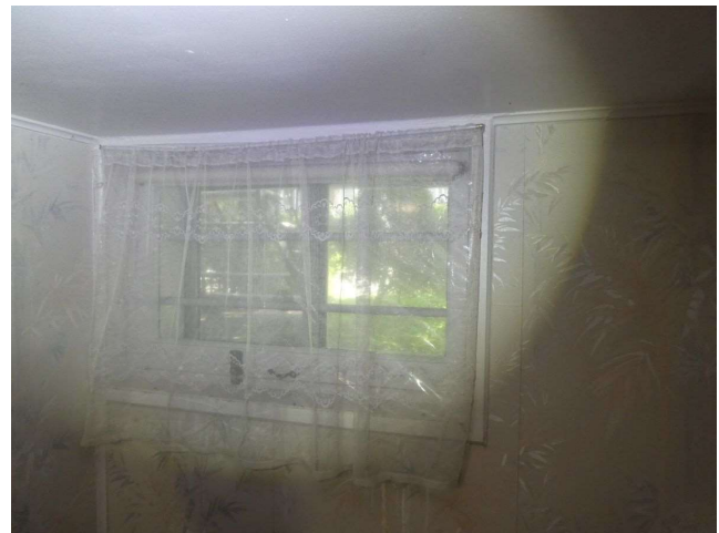
Basement (front room)
