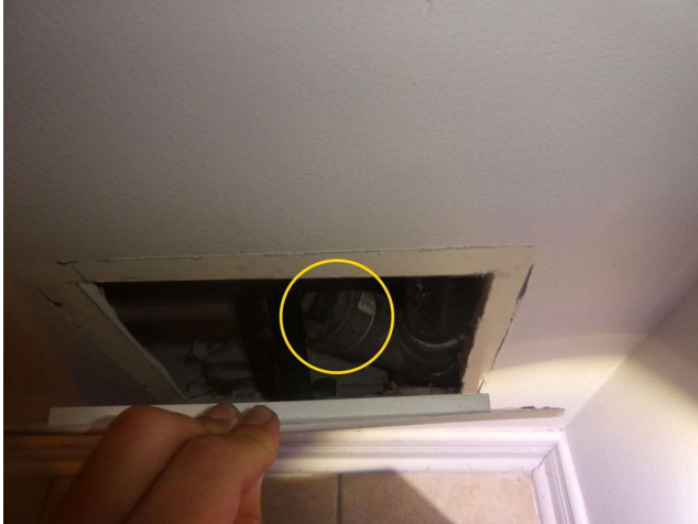
Mechanical room (exterior wall)
